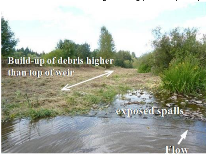
Southwest Channel Following Trimming (From Atop Weir)
