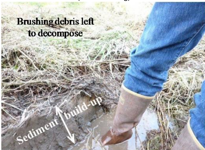
Sediment Build-up In Southwest Channel – 9/2010 (Post Trimming)
