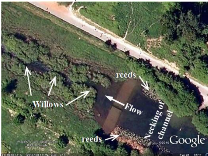
Recent Aerial Photo at Weir Showing Willow Overgrowth and Upstream Constraints
