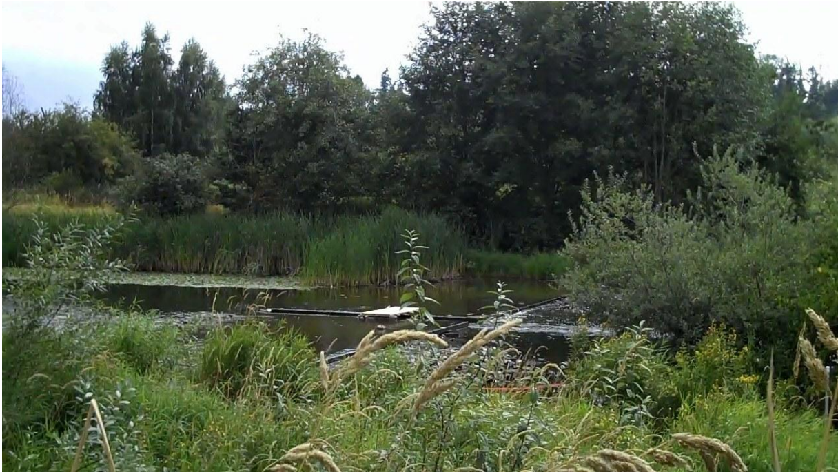
Figure 1 – Sammamish River Weir Prior to Trimming
