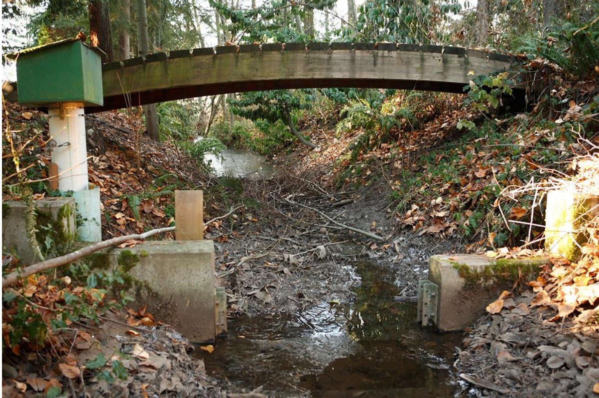
Figure 2 – Phantom Lake Outlet & Weir Prior to Cleaning
