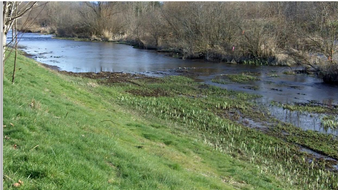
Obstructions and Sediment in Slough at Marymoor Park - March 2015
