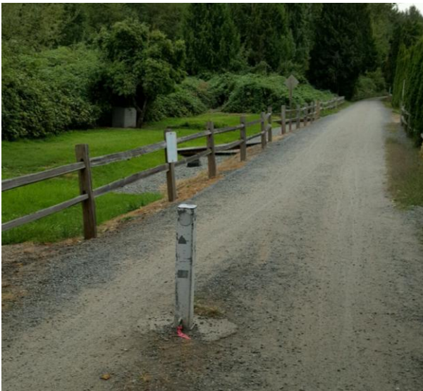
Trail Prior to Reconstruction
