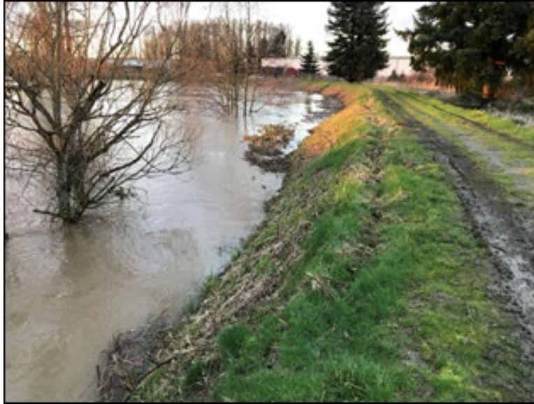
McCoy Levee on the Green/Duwamish River in Kent, 2021
