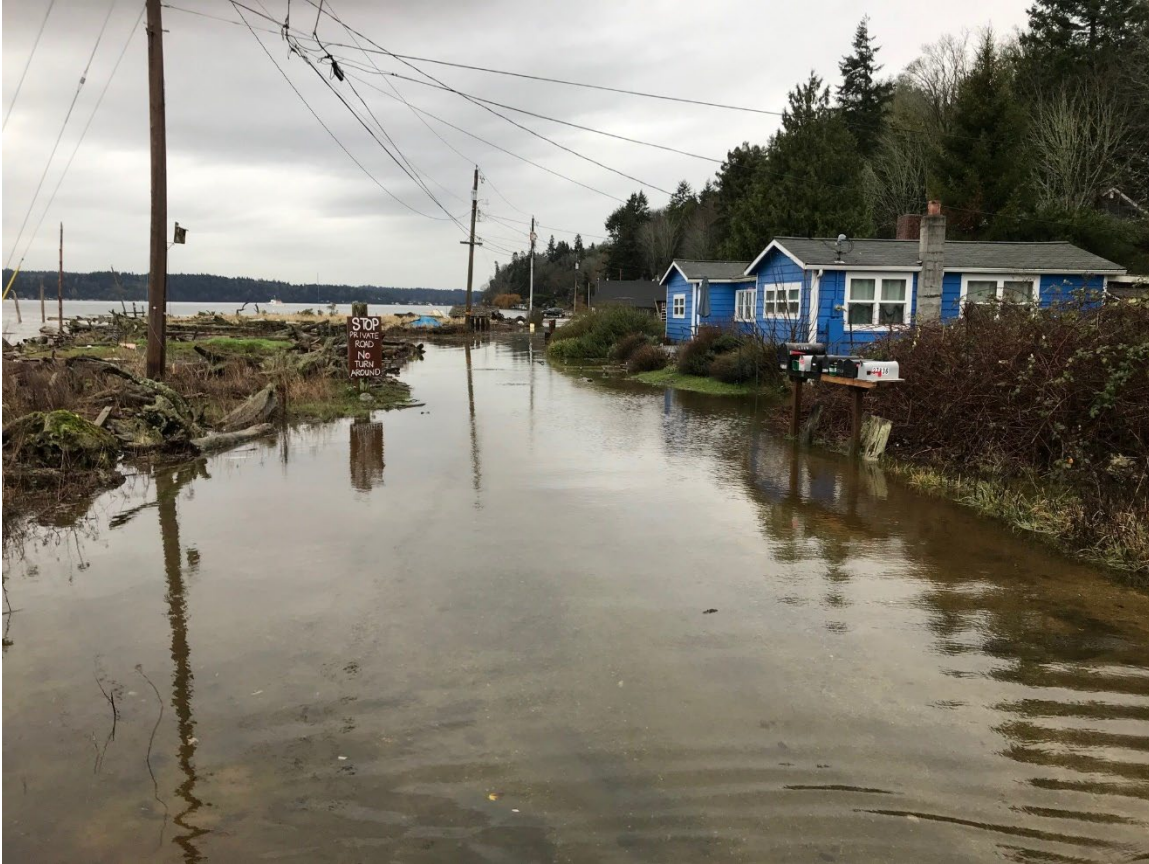
Waterfront road flooding on Maury Island, December 2022
