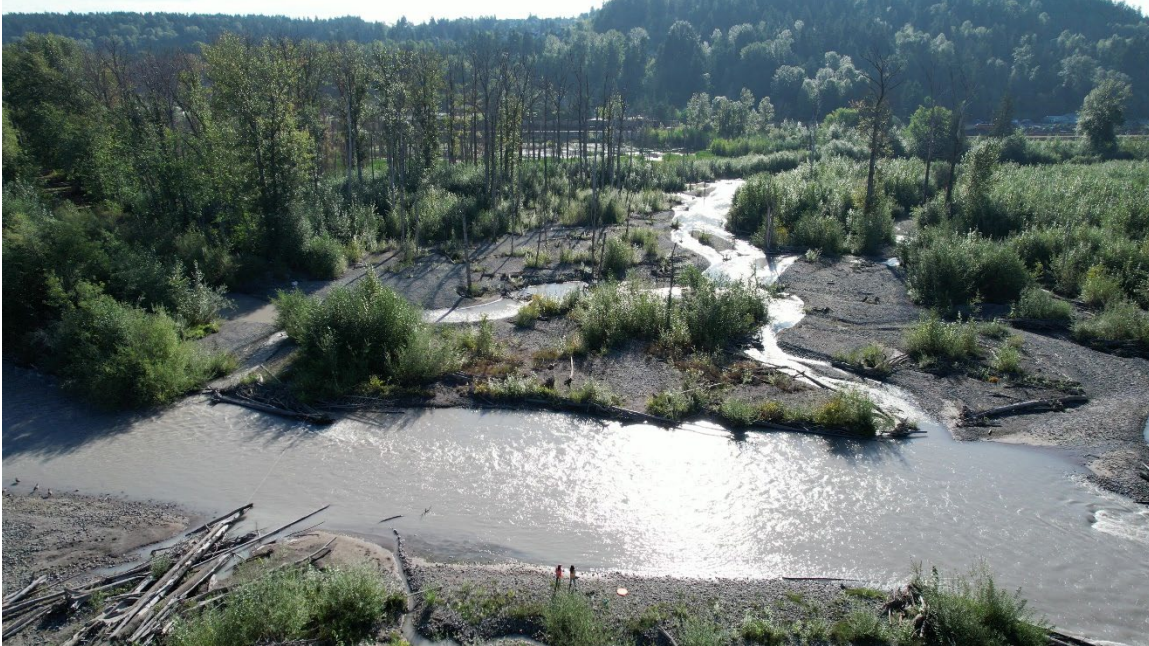
White River Countyline Floodplain Reconnection project, September 2023
