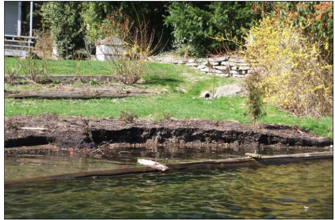
Figures 3a - 3d - Example Consequences of Misuse of Soft Stabilization
